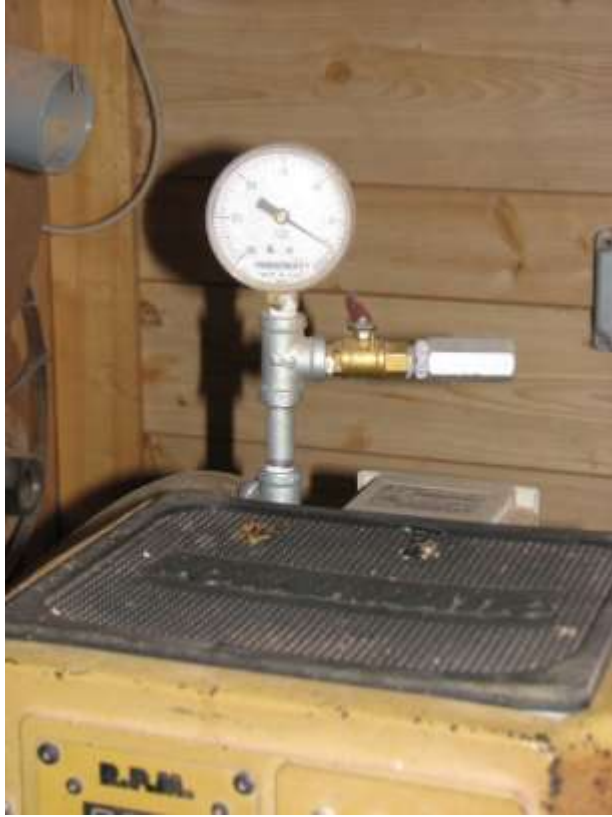
5 Placement for gauge and valve
